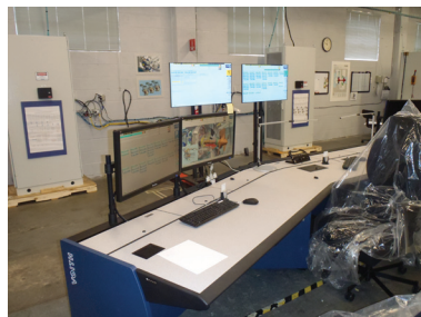
Staff members from AMP and Hamilton were on hand for the first week of testing of the Plant Control Switchboard (PCS). Testing will continue for another six weeks to verify controls are working properly.
